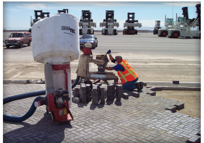
Figure 8. Saw cutting pavers.
