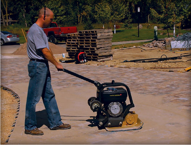
Figure 11. Vibrating sand into the joints.
