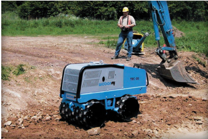
Figure 2. Compacting the soil subgrade.
