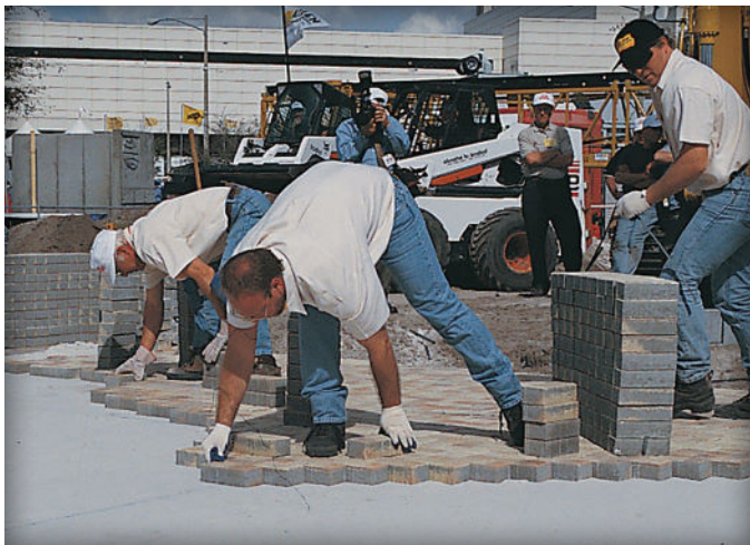
Figure 7. Placing the concrete pavers.
