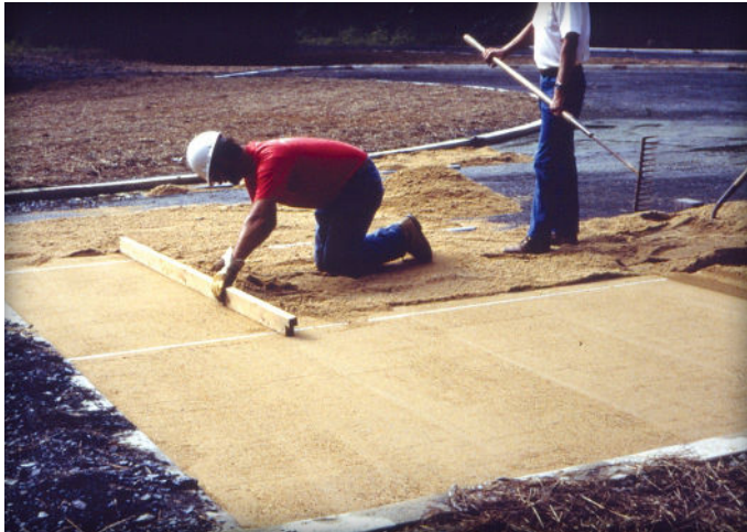
Figure 6a & 6b. Screeding the bedding sand.
