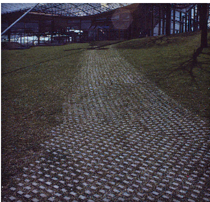
Figure 6. Service access lane
