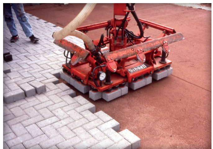
Figure 6. The vacuum head over the paver layer.
