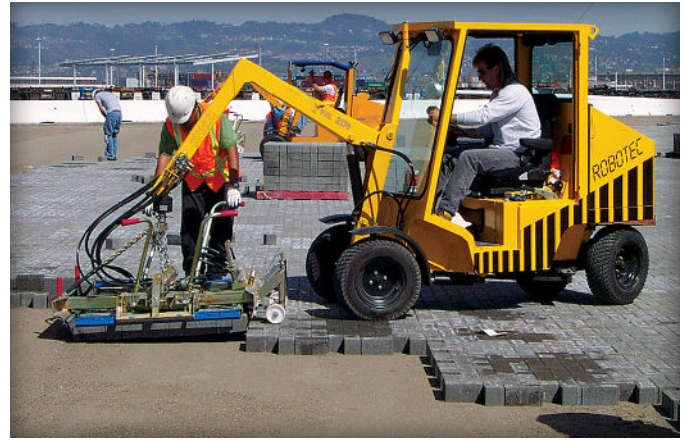
Figure 4. Hydraulic clamp picking up layer of pavers
